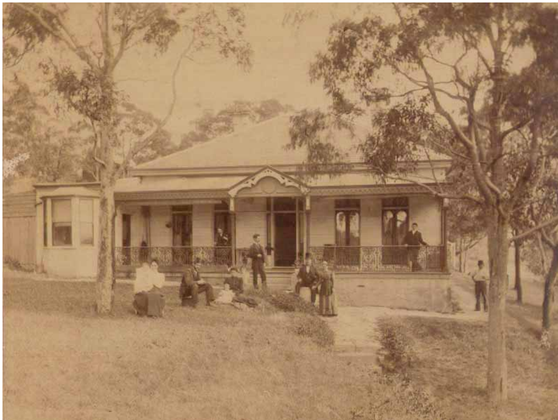
('Arden Lea' circa 1893, photo courtesy of Hunters Hill Historical Society and City of Ryde)
