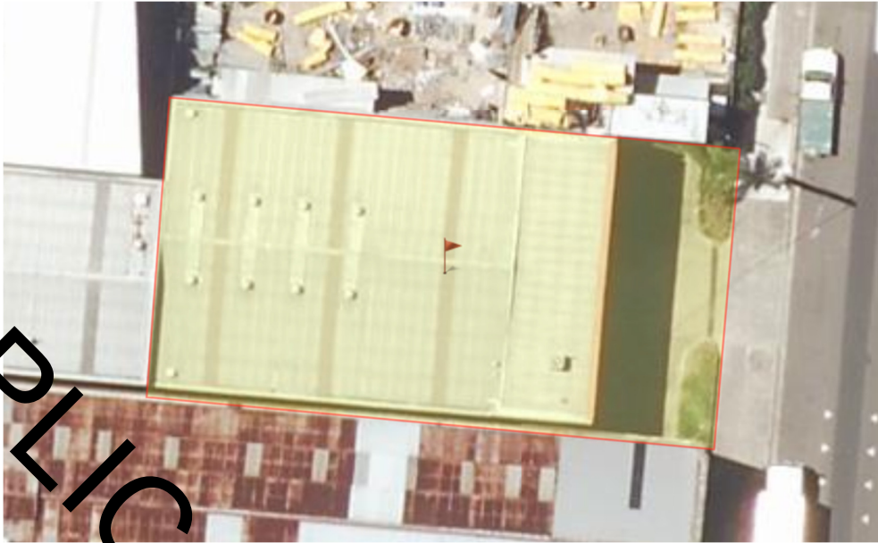
Figure 2- Aerial image of 10 Loftus Street, Turrella, as highlighted in yellow. Source: maps.six.gov.au
