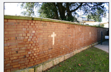
Heritage wall at Tempe House.
