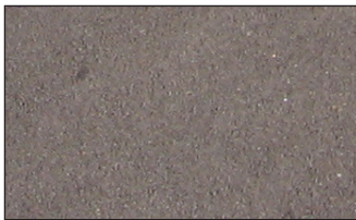
Asphaltic concrete paving
