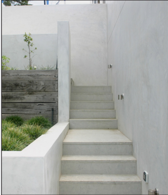
In-situ concrete steps
