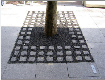
Paving units in Terrabond surface
