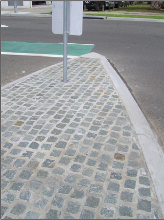
Central median- rumble strip
