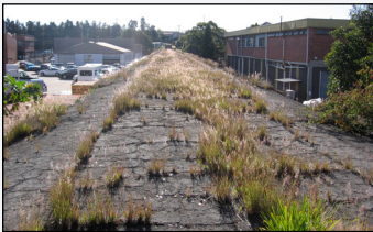
Plant colonisation along the SWSOOS
