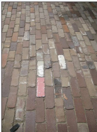
Recycled brick feature paving, Jacaranda Square.
