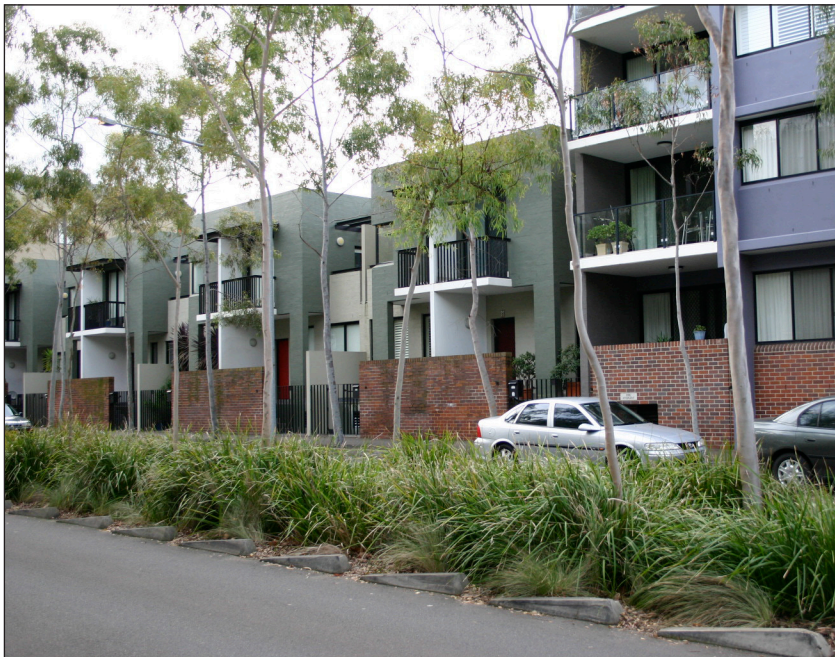
Central road swales
