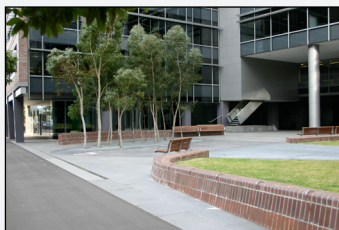
Level changes and brick wall seating.
