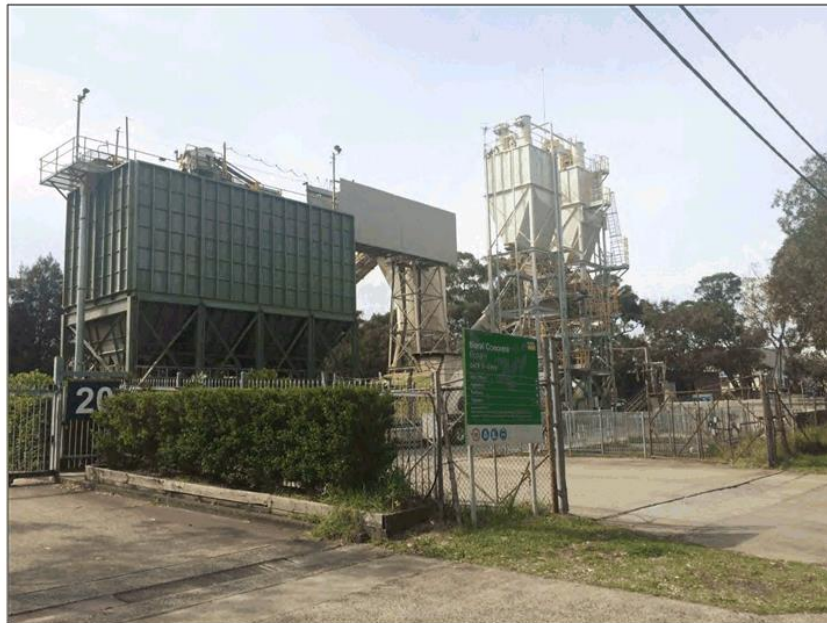
Plate 3: View of the site from adjacent property at 20 Anderson Street.
