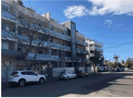
Figure 14: 284-290 Rocky Point Road, as viewed from Dillon Street
