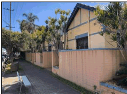
Figure 6: The subject site as viewed from Ramsgate Road
