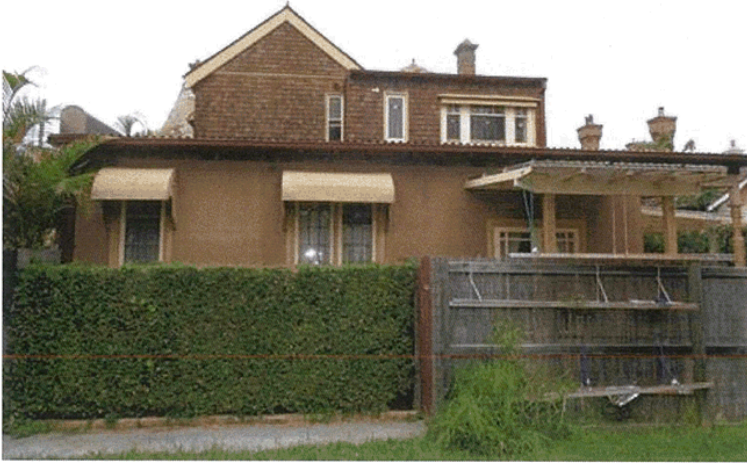
Figure 1 - Existing rear elevation. The ground floor windows will be filled in, the roof over the courtyard area will be removed and the new building attached at this point.
