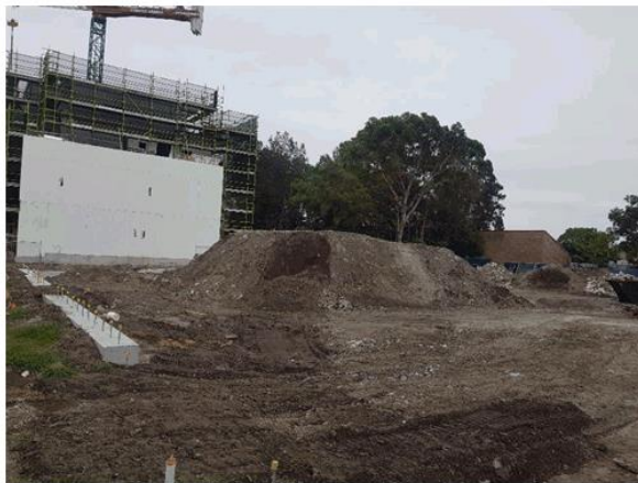
Figure 2: Looking towards adjoining development under construction at 27-29 Robey Street, Mascot
