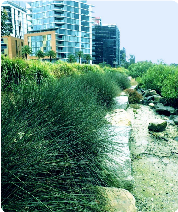
Cooks River Bank Restoration Works at Wolli Creek
