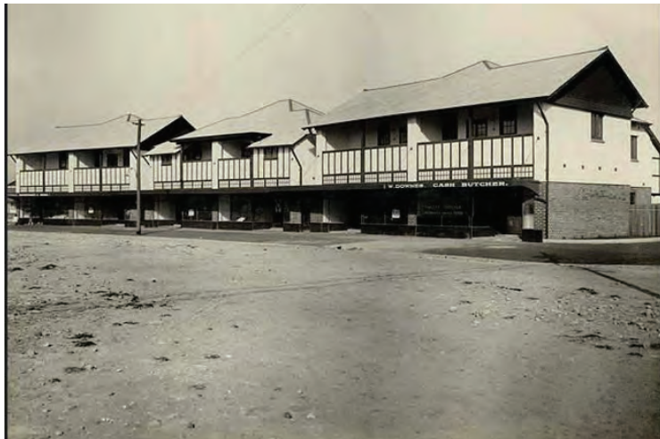
Fig.4.5.6 and 4.5.7 The theatre (top) and small group of shops (centre) were built at the commencement of the project, but most of the other planned community services and infrastructure, including a maternity hospital, technical college, four churches and a total of 40 shops were not pursued when the project was significantly reduced in scope in the 1920s. (NSW State Records)
