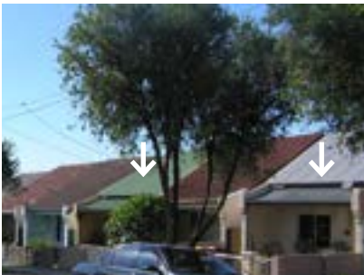
Example showing original separate verandah roof retained, Gibbs Street, Banksia
