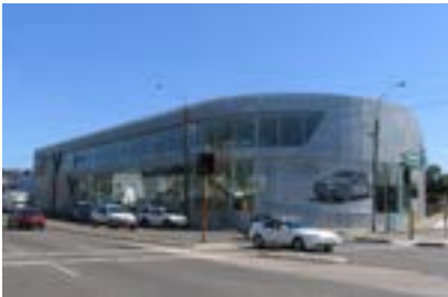
Example of commercial development along highways
