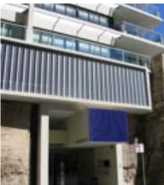
Building entries are clearly defined
