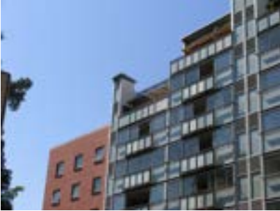
Loggias provide protection from road noise
