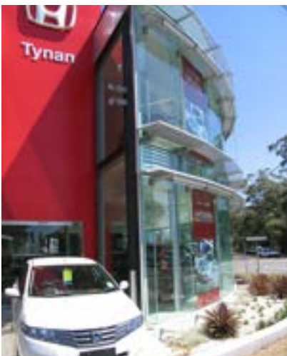
Environmental control devices add interest to facade design and protect glazing
