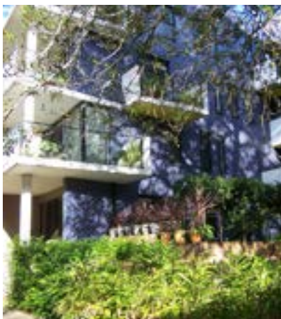
Balconies can provide quality open space and extend the living space of units
