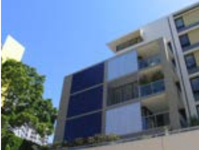
Operable louvres provide climate control
