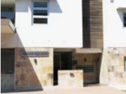
Letter boxes located in covered area adjacent to building entry
