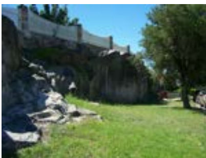
Sandstone walling and rock outcrop
