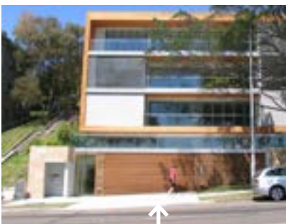
Garage doors are integrated with the streetscape
