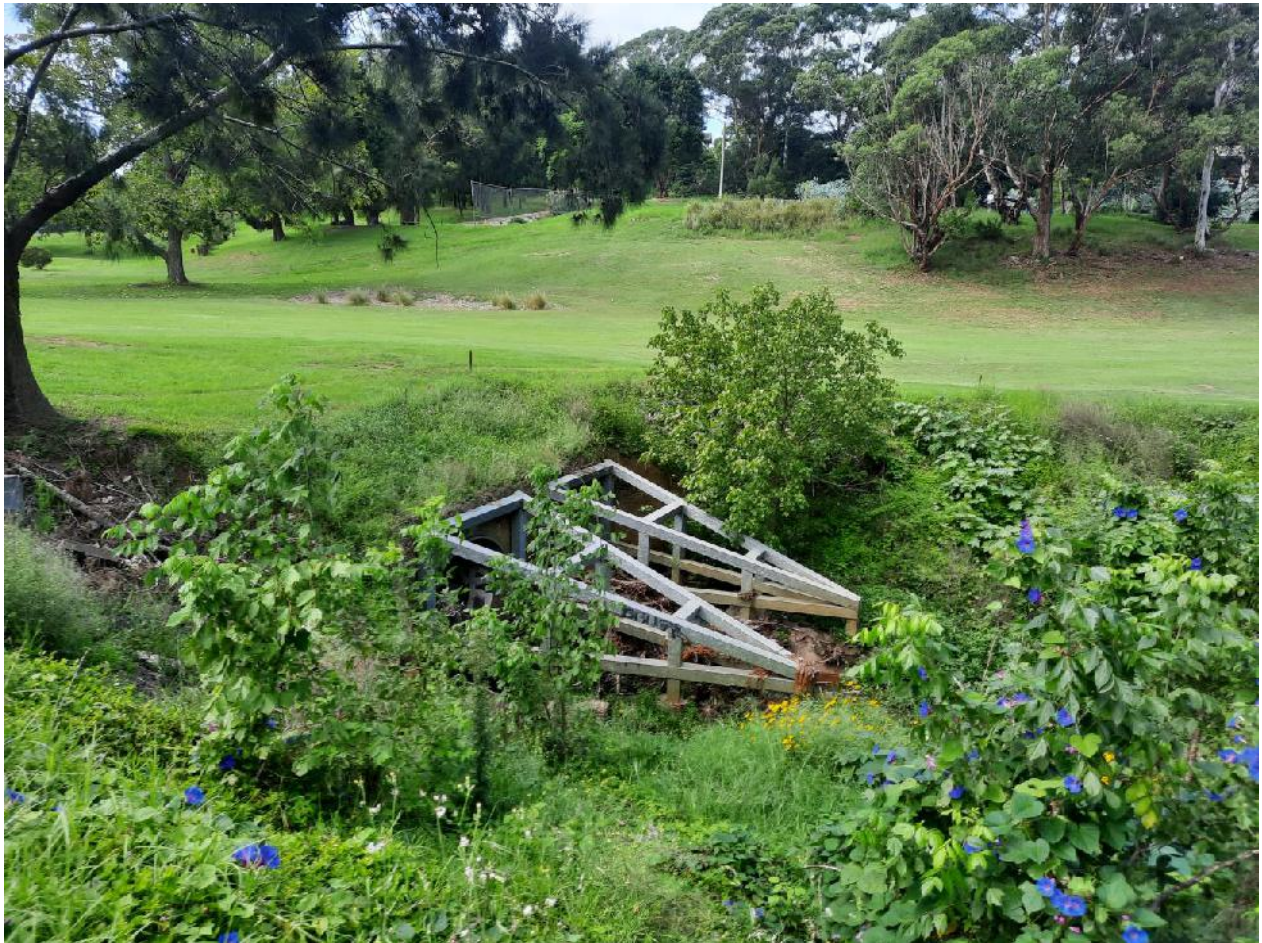
Photo 10: Bardwell Valley Golf Course Culverts
