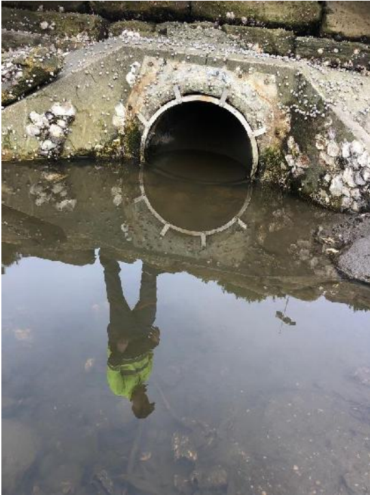
Photo 24: Inline non-return valve on a Cahill Park outlet to the Cooks River (Source: Bayside Council )
