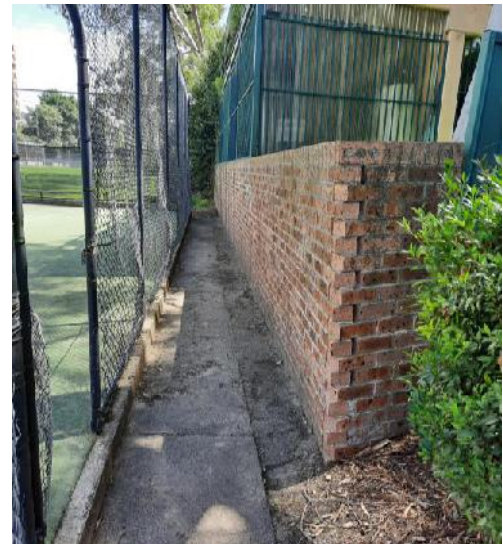
Photo 5: The Strand Levee wall
