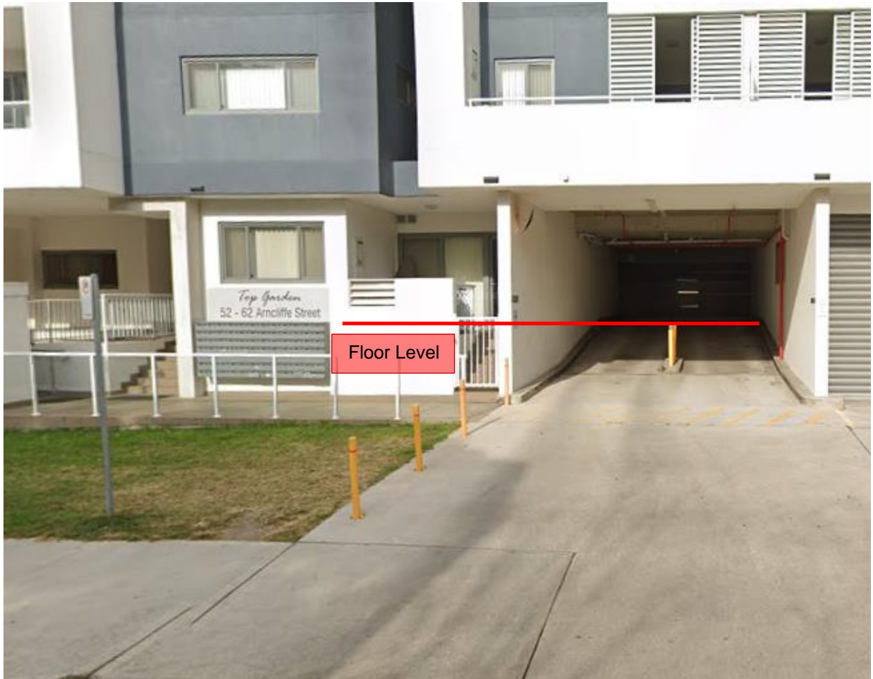
Photo 22: Typical apartment redevelopment on Arncliffe Street, with high floor levels and garage entrance crest levels ( Image: Google Street View )
