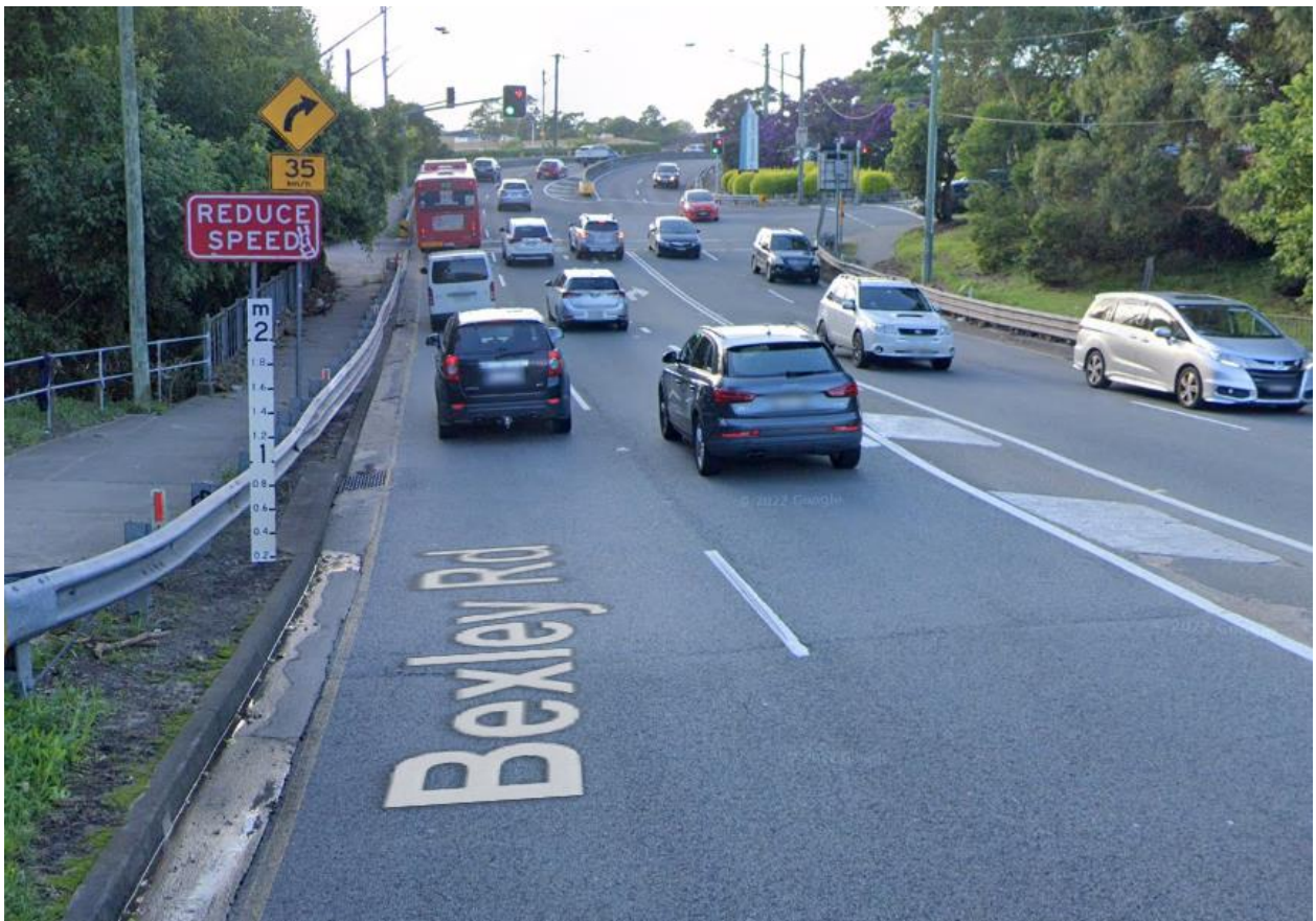
Photo 27: Flood depth indicator on Bexley Road crossing Wolli Creek (Image: Google Street View)
