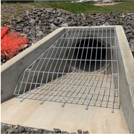
Photo 15: Example of a sloped culvert screen Image Source: https://australianmade.com.au/licenses/ej/gms-headwall--box-culvert-screens
