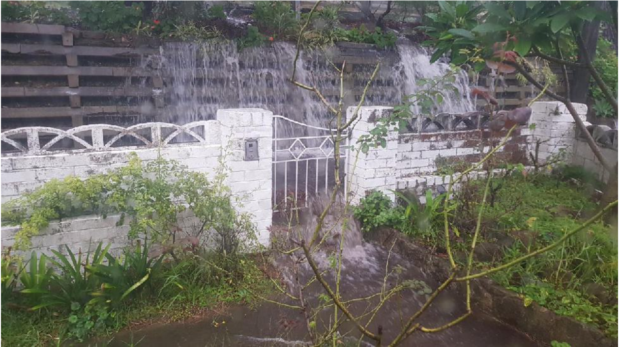
Photo 13: Water overtopping Kingsland Road at No. 17 during the February 2021 storms ( Image Source: Kingsland Road South Resident )
