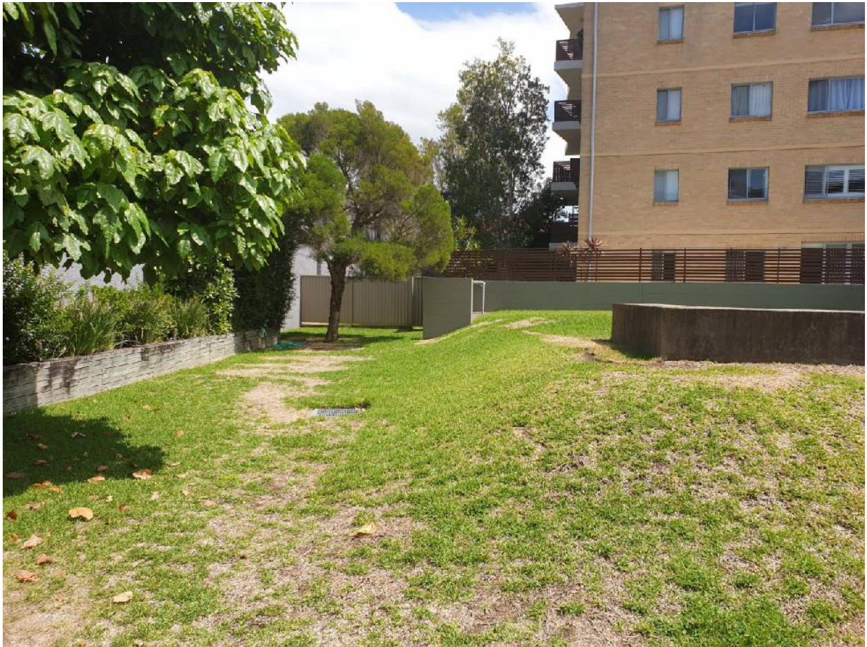
Photo 7: Development at 9 Banksia Avenue with a solid wall obstructing an overland flow path on the left
