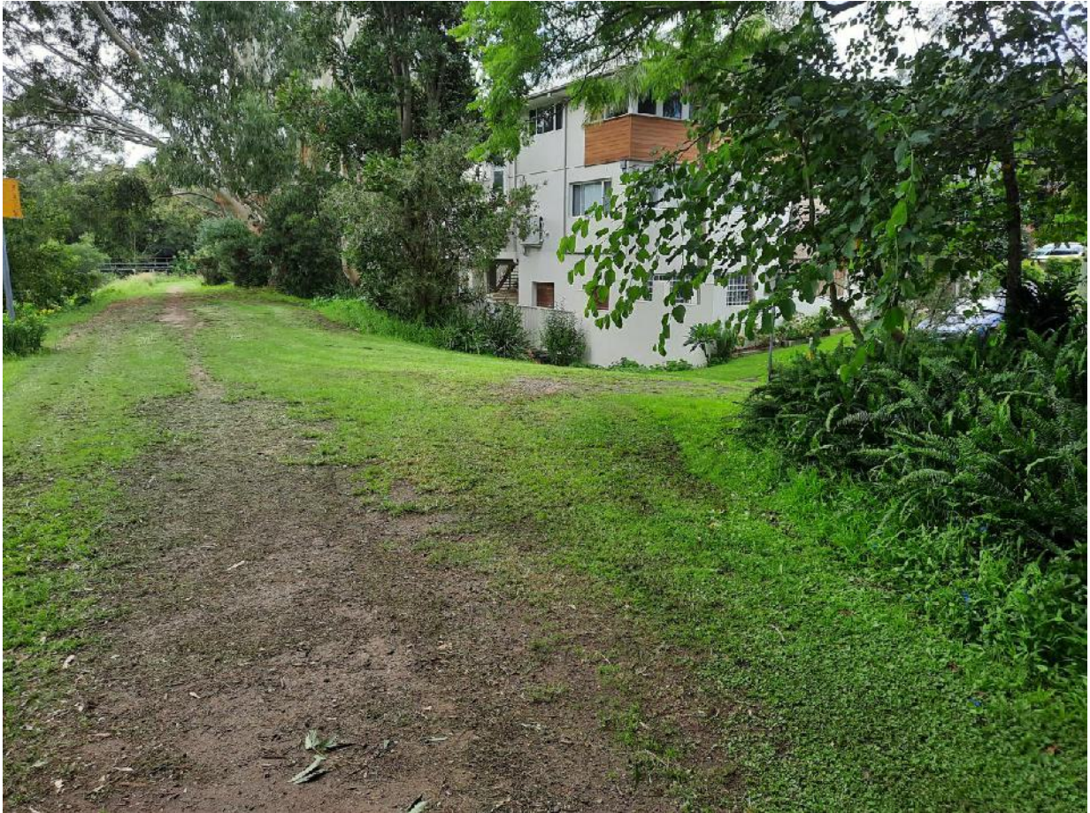
Photo 6: Hillcrest Avenue levee
