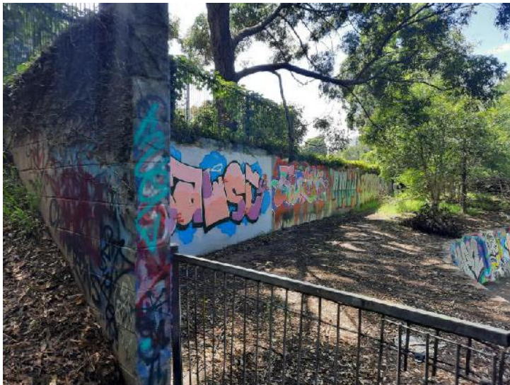
Photo 4: Frys Reserve Detention Basin wall
