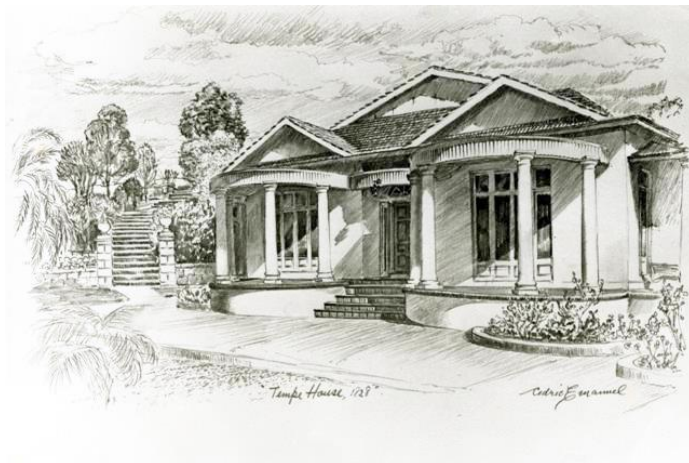
Tempe House 1828 Emanuel, Cedric, drawing, Image: Geeves, Philip, Sydney. Drawings by Cedric Emanuel, Angus and Robertson Pty Ltd, 1981
