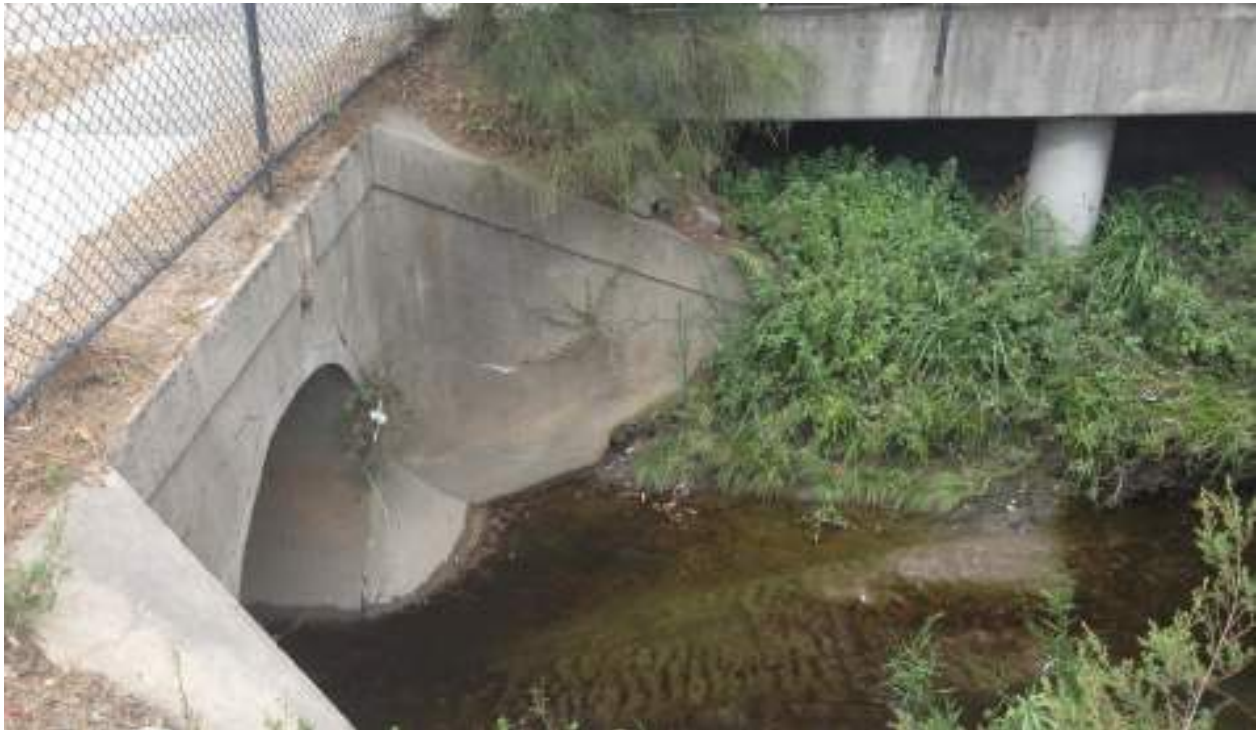
Photo 2 Existing 1800mm Floodvale Drain Culvert under Botany Rd
