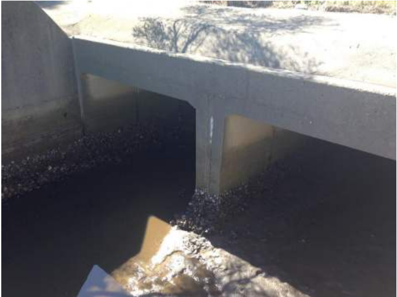
Photo 3 Floodvale Drain outlet downstream of Foreshore Road
