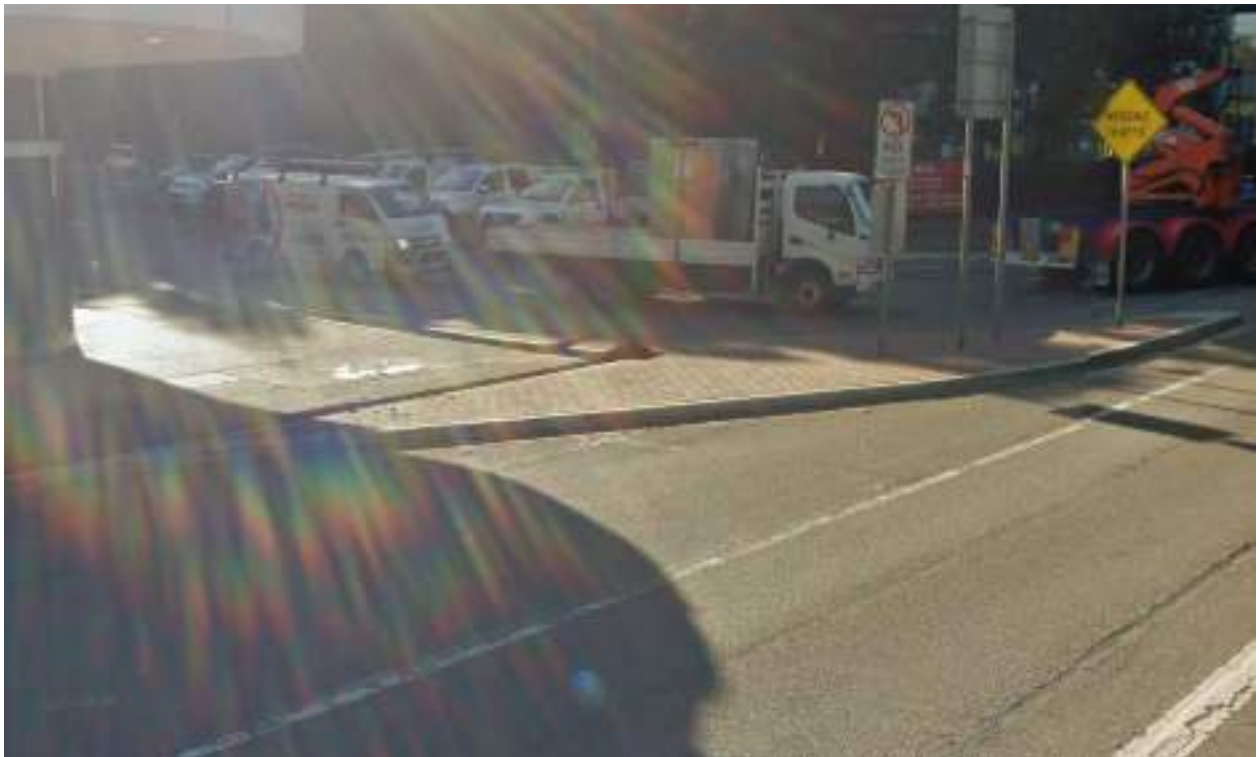
Photo 9 Sag point at corner of Exell Street and Botany Road
