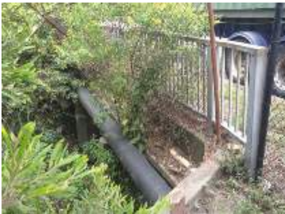
Photo 4 Springvale Drain culvert under McPherson St (downstream end)
