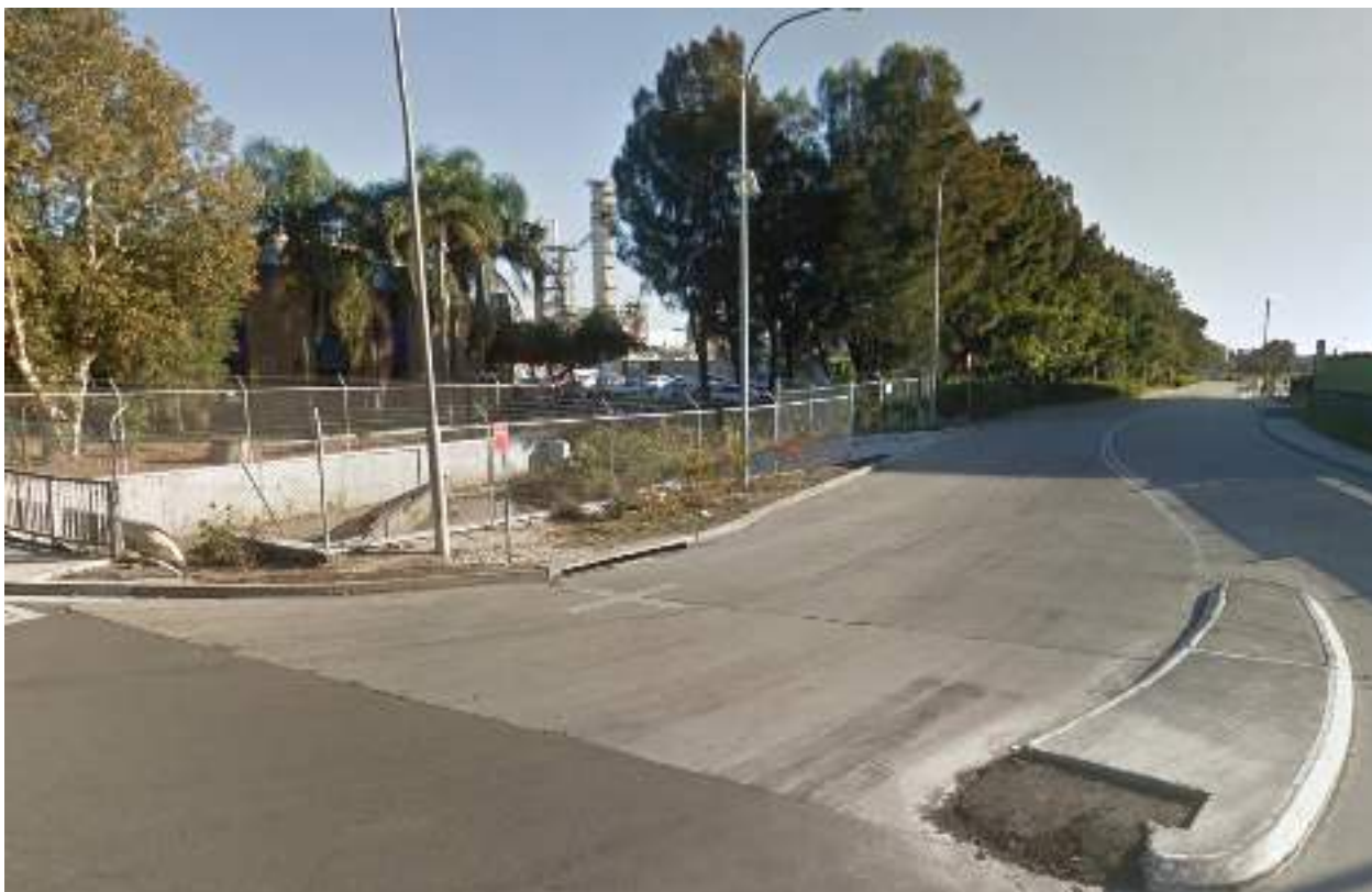
Photo 10 Sag point at corner of Coal Pier Road and McPherson Street
