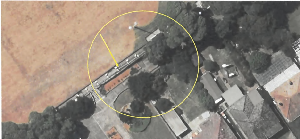
Figure 2 | Aerial of Gardiner Park indicating up with the approximate location of the collapsed wall for repair. [SIX Maps]
