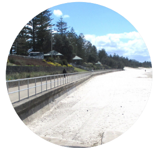
Promenade seawall along beach
