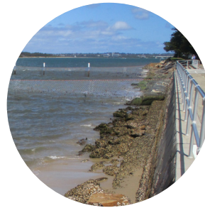
Hard sea-wall shoreline
