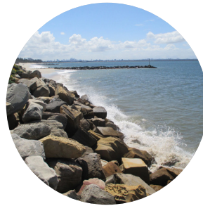
Rock protection at Emmaline St
