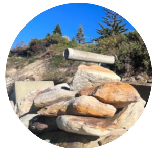
Repairing damaged infrastructure
