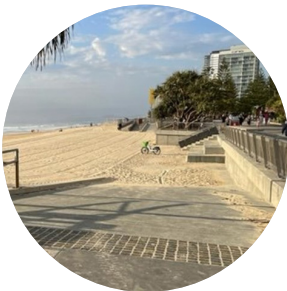
Equitable beach access & seawall upgrades Surfers Paradise, QLD; Accessible Beaches
