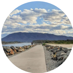
Groyne upgrades North Haven Breakwater, Port Macquarie Hastings Council
