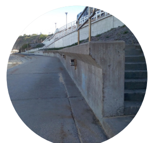
Seawall maintenance and upgrades Newcastle Beach, NSW
