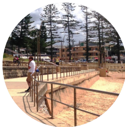
Seawall maintenance and upgrades Dee Why, NSW Weekend Notes
