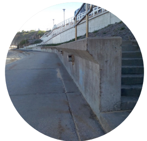
Seawall maintenance and upgrades Newcastle Beach, NSW
