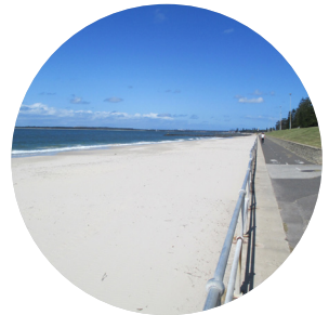
Promenade seawall along beach
