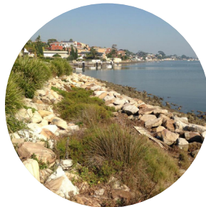
Eco-friendly seawall adaptation Intertidal saltmarsh seawall Claydon Reserve, NSW
