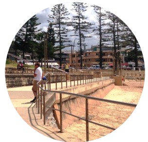
Seawall maintenance and upgrades Dee Why, NSW; Weekend Notes
