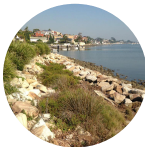
Eco-friendly seawalls Intertidal saltmarsh seawall, Claydon Reserve, NSW OEH 2009
