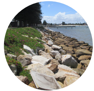
Lena Street Rock Revetment
