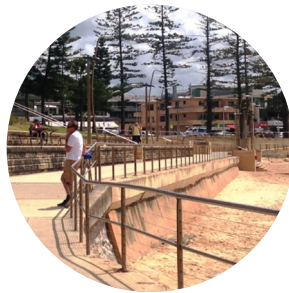
Seawall and groyne upgrades
